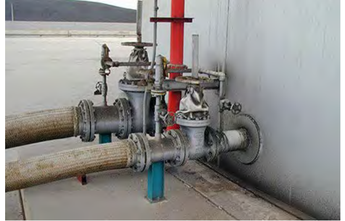
Fig. 2.17.6 > Raccords flexibles
